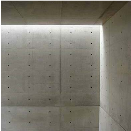
7. OFF FORM CONCRETE
